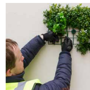
STEP 6 Re-adjust any plants on the cut parts and fill in all the gaps with loose foliage.
