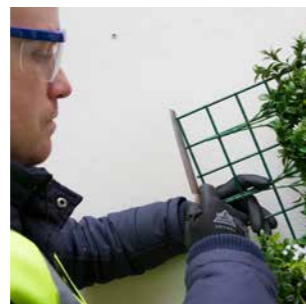
STEP 3 File the grid after cutting.
