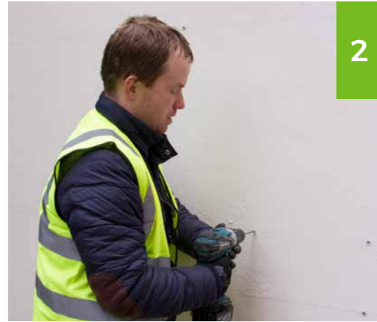
Drill the holes
