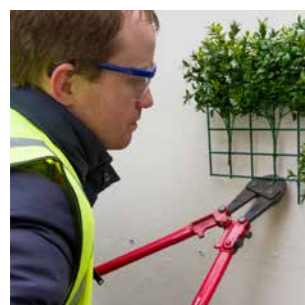
STEP 2 Clip off the excess as close as possible to a grid section and separate the parts.
