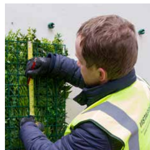
STEP 1 Measure carefully and mark the area to be trimmed.
