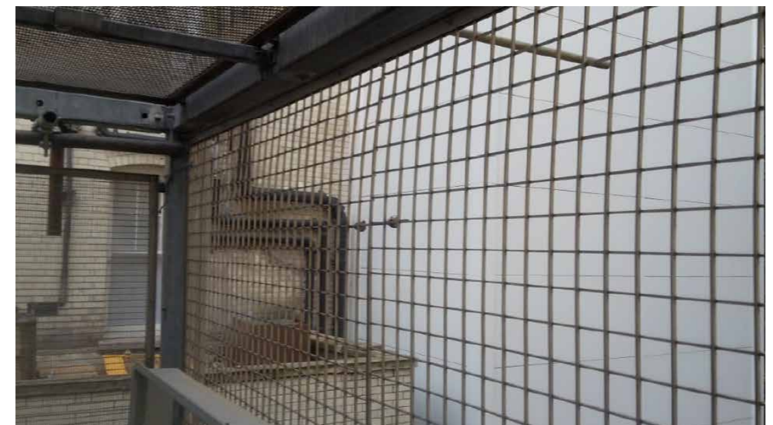
Metal cage before Vistafolia® Panel installation
