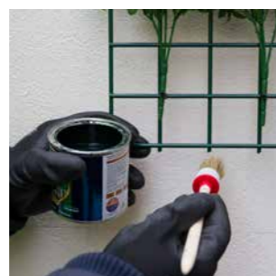
STEP 4 Protect cut point with metal paint.
