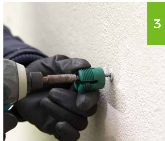
Plug & screw the fixing
